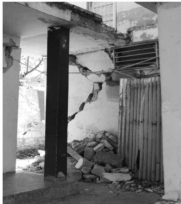
One of many devastated buildings in Port-au-Prince, Haiti, following the mid-January earthquake.
